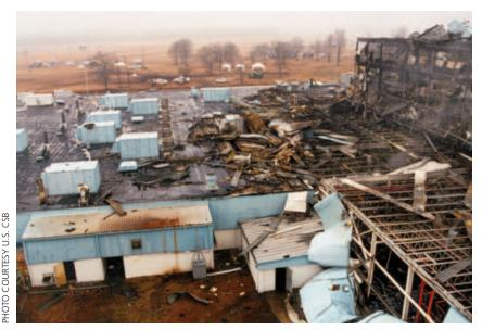
West Pharmaceutical Services, Kinston, NC, January 29, 2003. Six people lost their lives, and 38 were injured. dust. Now imagine that same energy release in a confined space such as a machine or building. The pressure wave from the rapid burning of the dust cloud tries to expand quickly. The vessel contains the pressure and allows it to build until it rapidly bursts out of its confinement. This is typically called a dust explosion.
