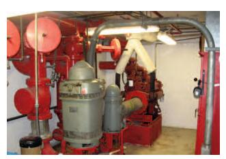
Photo 5: Two vertical turbine fire pumps taking suction from a reservoir. The pump room floor is the top of the water reservoir. The near unit has an electric motor mounted vertically on the pump. Behind is a diesel driven vertical turbine pump with a right-angle drive.
