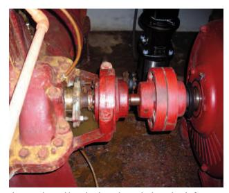
Photo 4: The packing glands are located where the shaft enters the pump. The inboard bearing is on the pump housing frame. The flexible coupling is located between the pump and the driver.
