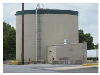
Photo 2: A fire pump house and suction tank. Note the fire pump test header and fire department connection.
