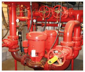
Photo 3: Two in-line fire pumps installed side by side in a pump room.
