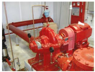
Photo 1: A typical electric fire pump installation. An electricdriven fire pump with the controller to the rear and the jockey pump to the left.
