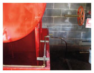
Photo 7: Diesel tanks must be at least 2/3 full. Valves should be within the containment area to help prevent leaks at the threads from spilling into the pump house. The author has seen improperly maintained pump houses with diesel fuel covering the floor to ½-in. in depth.
