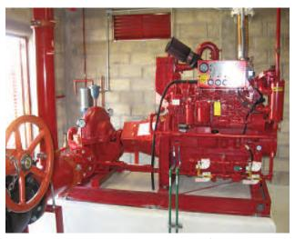
Photo 6: A diesel-driven horizontal split-case fire pump. The instrument panel is at the top of the engine. The cooling line and bypass are located alongside of the engine. The batteries are located on the opposite side of the engine so the operator does not stand in front of, or reach over them, to operate the pump.
