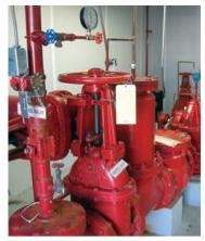
Fire pumps supply adequate pressure and volume for many fire supression systems. In this impairment, the pump's main discharge value is shut off.
